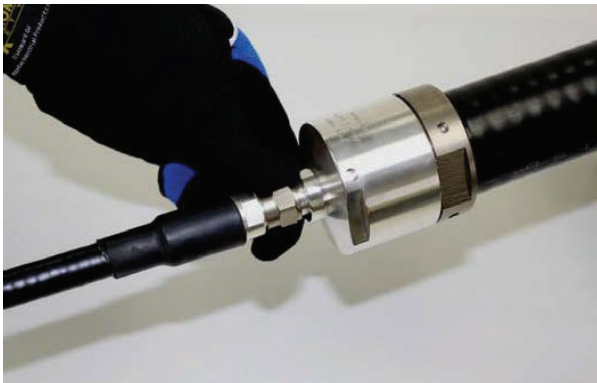
Step 1 - Attach coupler nut finger tight
