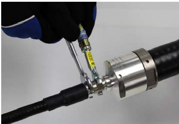
Step 3 - Use torque wrench to tighten coupler nut until the wrench handle "clicks", at this point the proper torque has been applied
